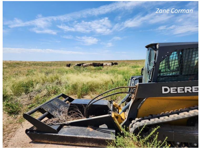
Figure 17. Skid steer outfitted with rotary cutter attachment.
