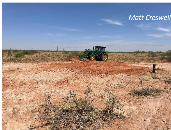
Figure 28. CEHMM staff preparing an old pad for reseeding.
